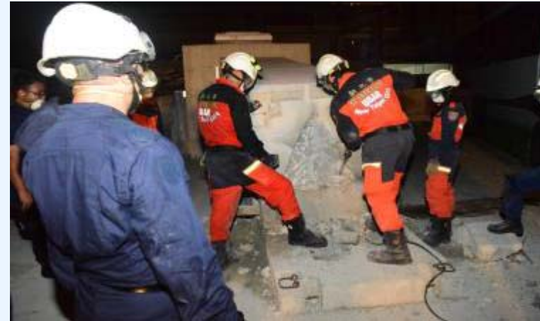
Conducting breaching to gain access
